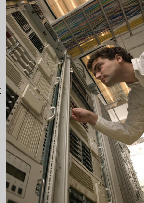
Orion Group Engineers have over 70 years experience operating in virtually every network environment
